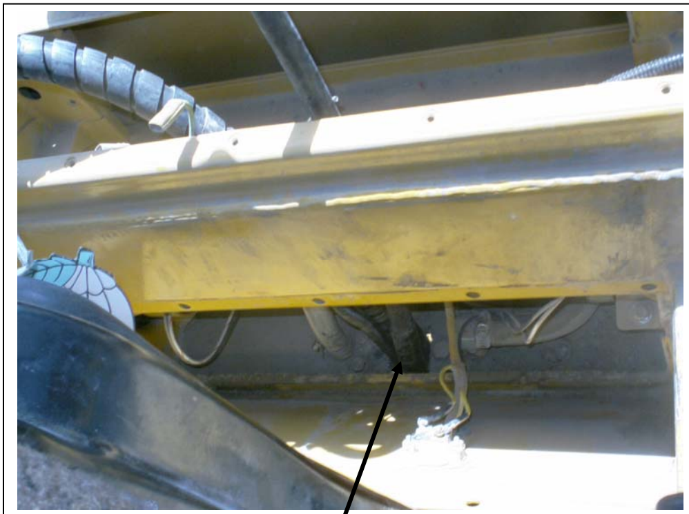
A/C hoses and wiring coming up through the floor of the cab.
