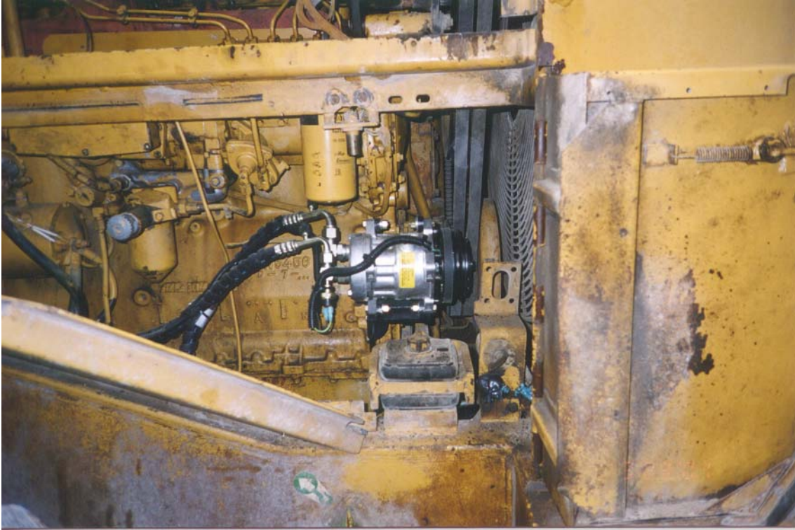
Compressor and mount in place.
